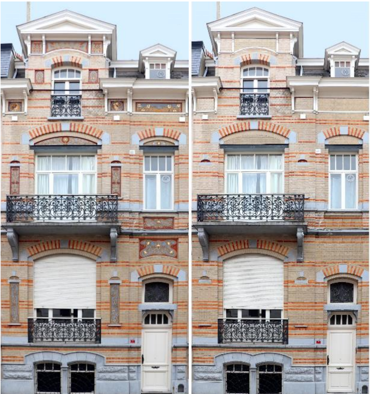
Rue Jenneval 15, Bruxelles Extension Est, 1902
